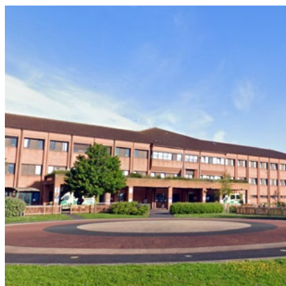
Musgrove Park Hospital, Somerset NHS Foundation Trust
